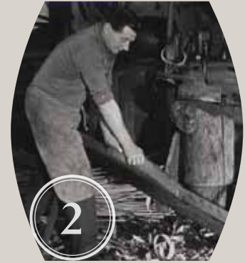
2 Smoothing the stave edges with the 'jointer' to create a neat marriage between neighbouring staves
