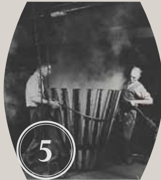
5 Pulling together the stave ends, whilst still soft, with a rope
