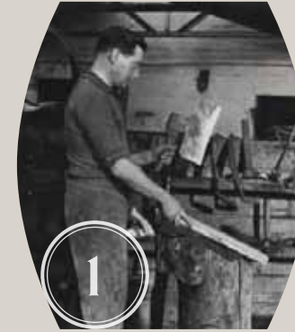
1 Using the 'axe' to roughly shape the staves, typically made from seasoned oak
