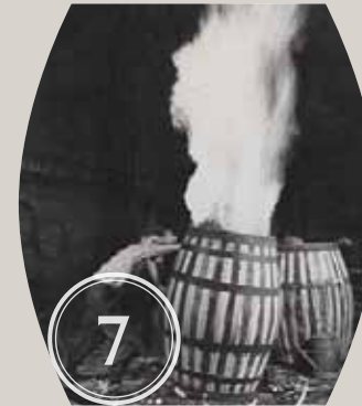
7 Charring the inside of the cask, by placing it over lit wood shavings, to dry and seal it
